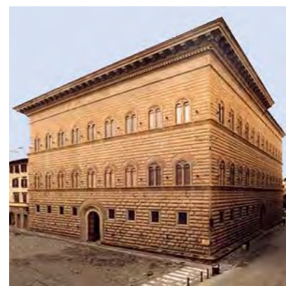
The first CU site beyond the UK was the Palazzo Strozzi in Florence
